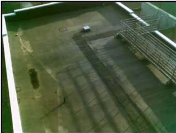
Figure 4: Photo of the South roof of IIHR.
